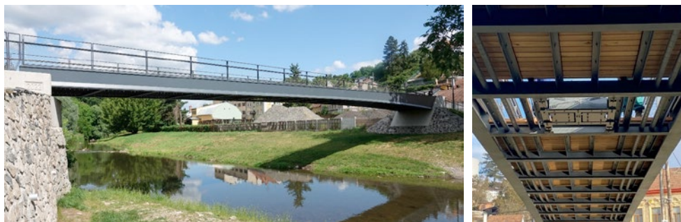
Figure 4 Footbridge over the Svitava River in Bílovice nad Svitavou, Czech Republic, equipped with a tuned mass damper KGF (Nečas, 2023)
